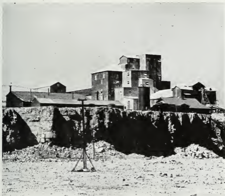
Huge quarries occur in the State that yield large tonnages and convert stone resources into wealth.
